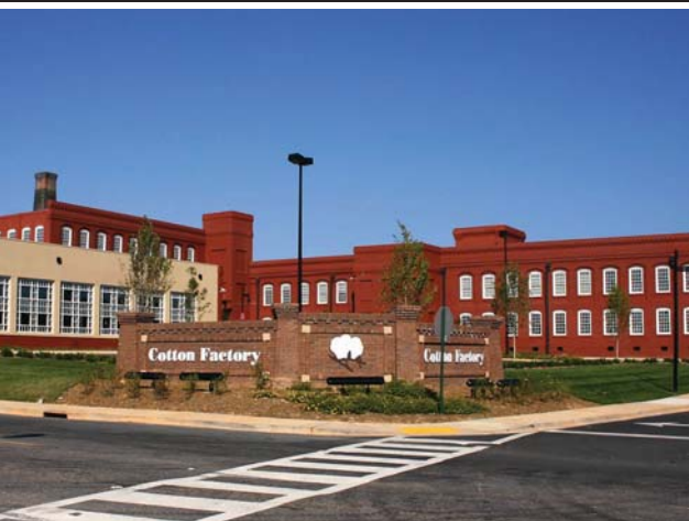
Left: The renovation of the Rock Hill's Cotton Factory marks the first major accomplishment of the Textile Corridor redevelopment plan to create a pedestrian-friendly, mixed-use, urban village in the former textile manufacturing area of the city.
