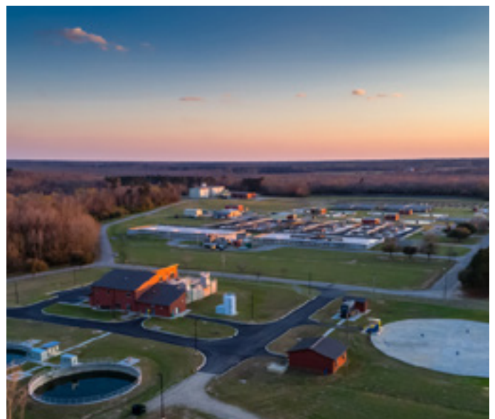
Sumter WTP No. 6
