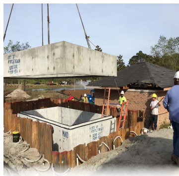
82nd Avenue North Pump Station, Myrtle Beach, SC - Wetwell Installation. Construction Services by DDC Engineers
