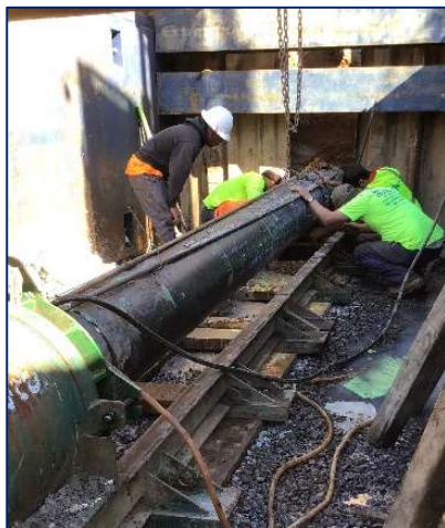
Figure 4 – Sewer Main Construction
