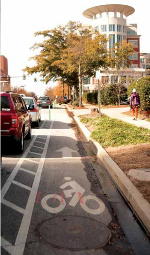
This bike lane on Broad Street in downtown Greenville uses parked cars to separate bicycles from car traffic. Photo: Michael Dantzler.
