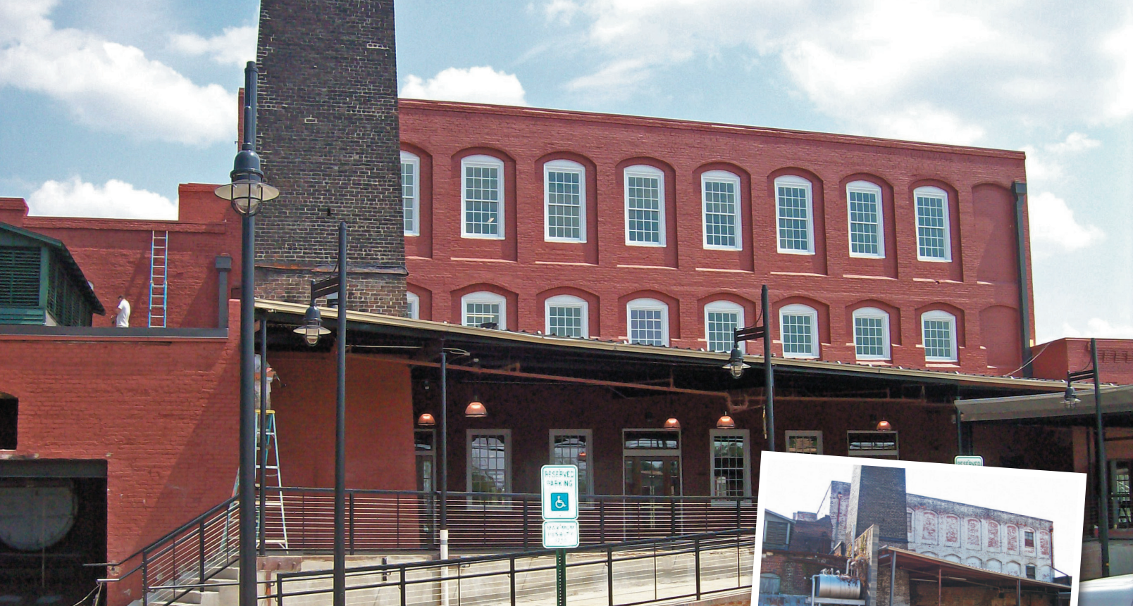
The renovation of the Rock Hill's Cotton Factory became an early success in Rock Hill's drive to redevelop the former textile manufacturing district of the city. Photos: City of Rock Hill.
