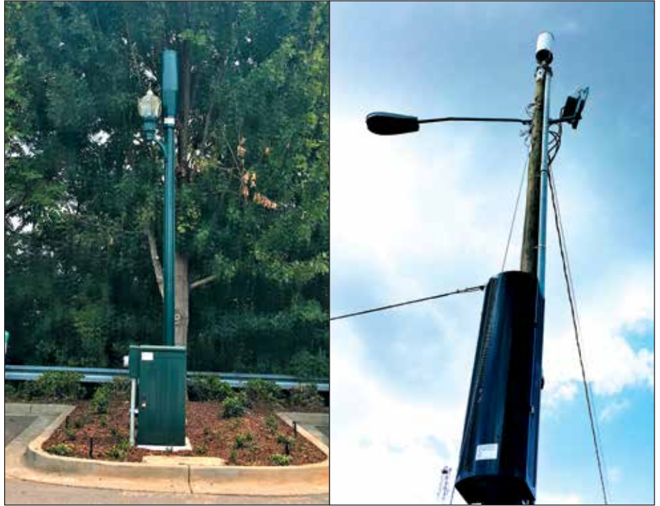
Small wireless facilities in the City of Columbia attach to telephone poles and other structures.
