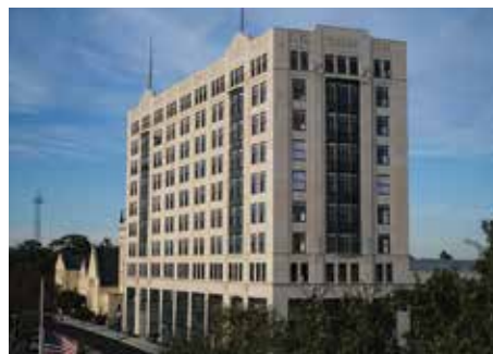
The redevelopment of the Montgomery Building has been a major topic of discussion in the redevelopment of downtown Spartanburg. Photo: City of Spartanburg.
