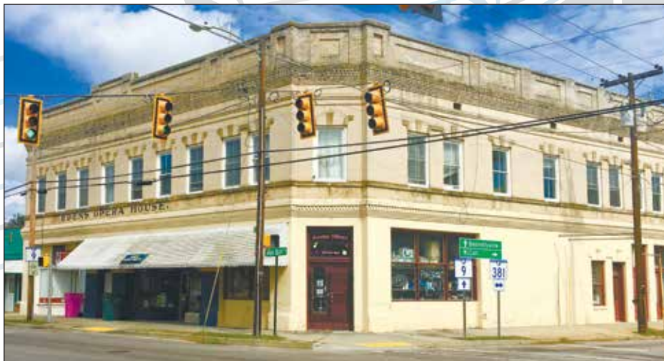
The Edens Opera House in Clio houses youth development groups, a church and an auto parts store. Photo: Town of Clio.
