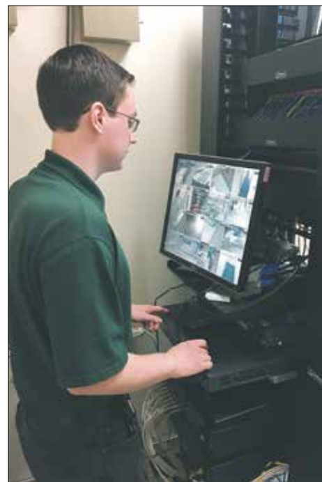
Jeremy Hirtle, IT technician, monitors the city’s facilities. Photo: City of Lancaster.
